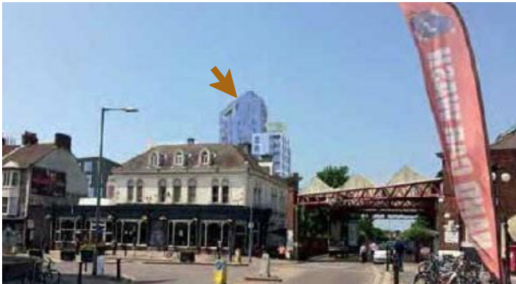
Figure 10 - Hove Gardens viewed from Goldstone Villas
