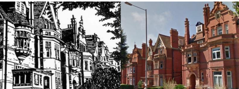
Figure 14 - The Drive Conservation Area
